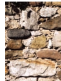
The villages round the hills were mostly built from local stone. This old wall in Falkland Library car-park contains a superb collection of rocks, held together with mortar probably made from Lomonds limestone.
